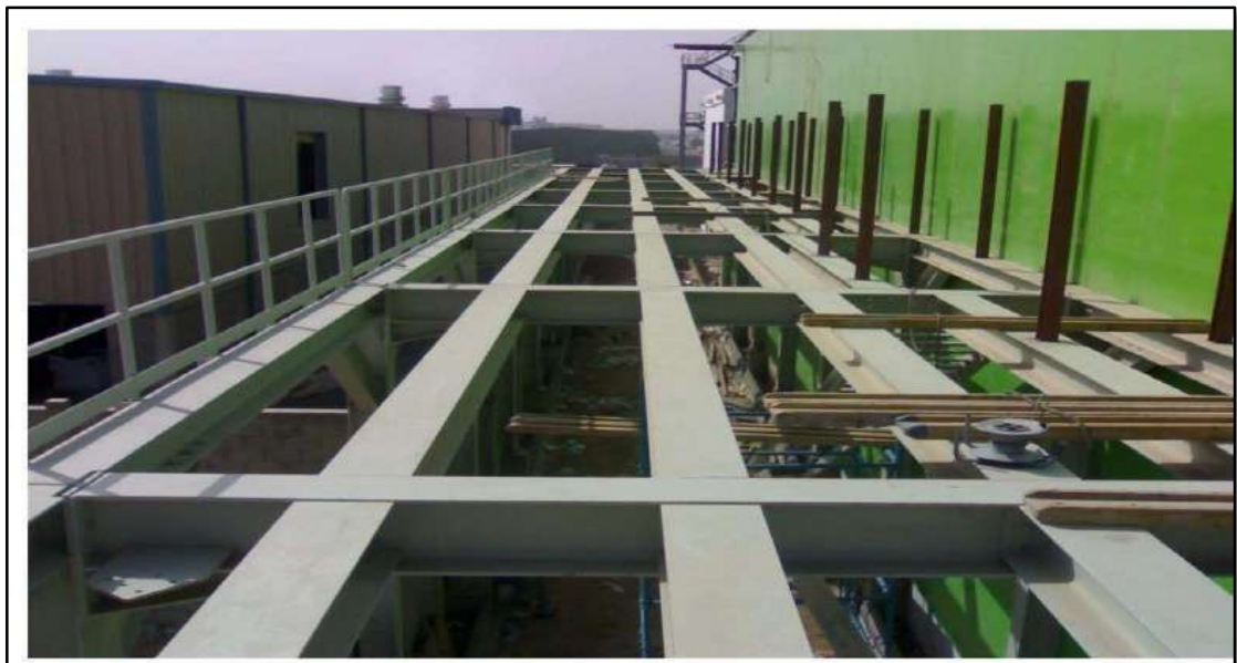
SUPPLY AND INSTALLATION OF CHILLER PLATFORM
