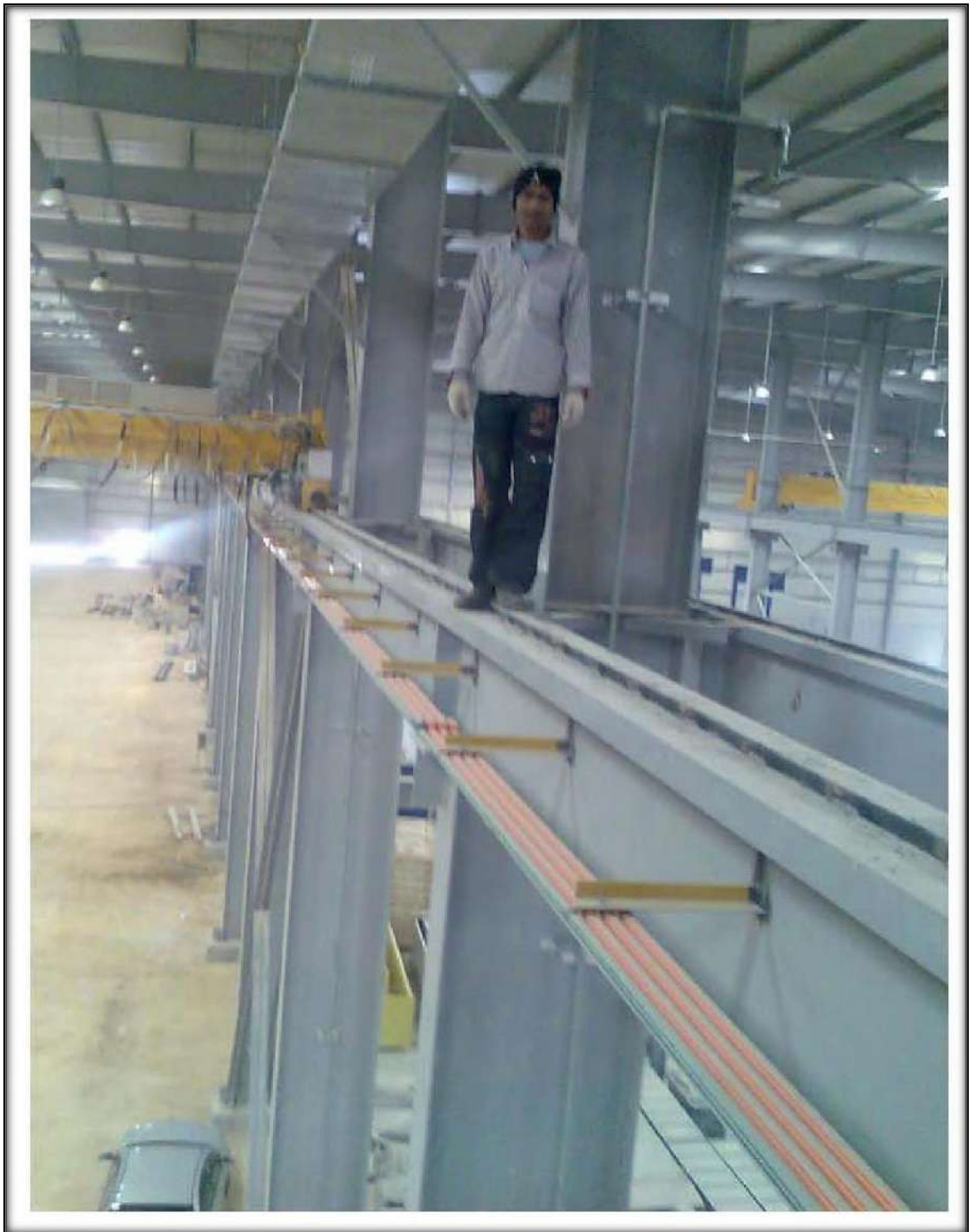
350M LONG STEEL STRUCTURE ERECTION AND CRANE BEAMS INSTALLATION LOCATION: INDUSTRIAL DUCTILE IRON PIPE COMPANY (INDIPCO) - JUBAIL
