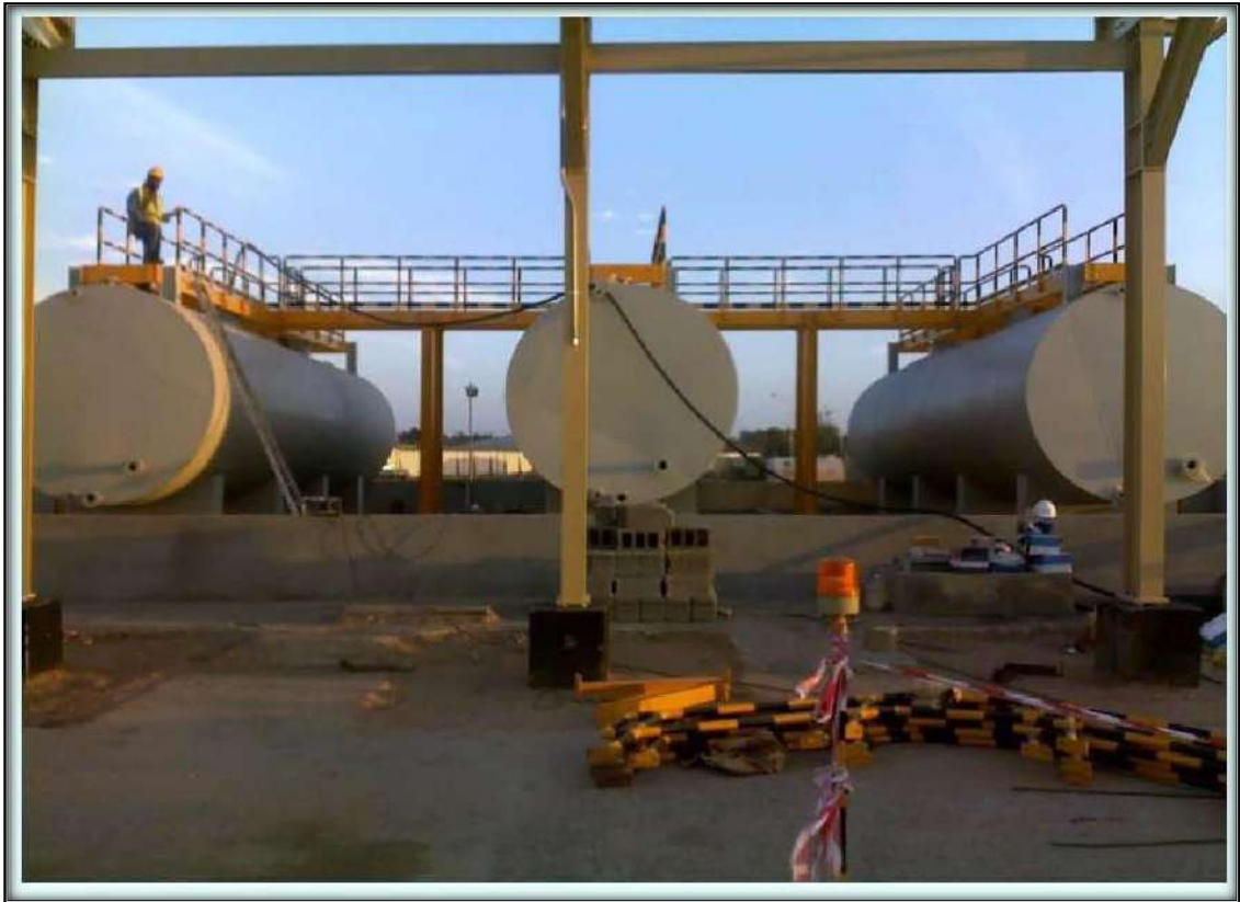
SUPPLY AND INSTALLATION OF JET FUEL OIL TANK AND CATWALK
